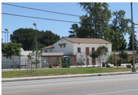
Current Pool House, recently restored awaiting addition of the new pool.
